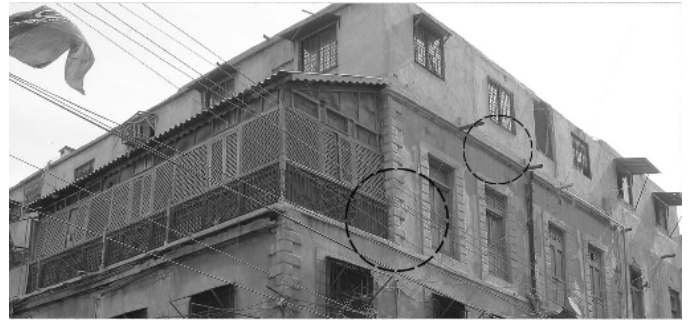
This heritage building exhibits the attachment of a pol house extension with the limestone brick quoins, and the attachment that the concrete vertical encroachment has with the roof slab
