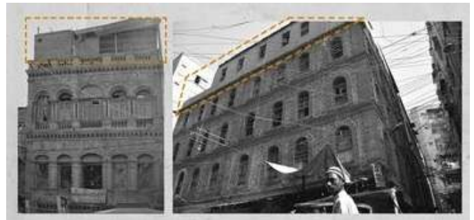
The top building articulation of the heritage building/modern building exhibits a make-shift extension. These encroachments are hardly completed installations, still in their construction phase and lacking a finishing plaster for their brick walls. The walls and floors are basically cemented onto the limestone facade/roof on top for additional reinforcement in terms of structural integrity e.g. as we see in the Haji Hashim Building.
