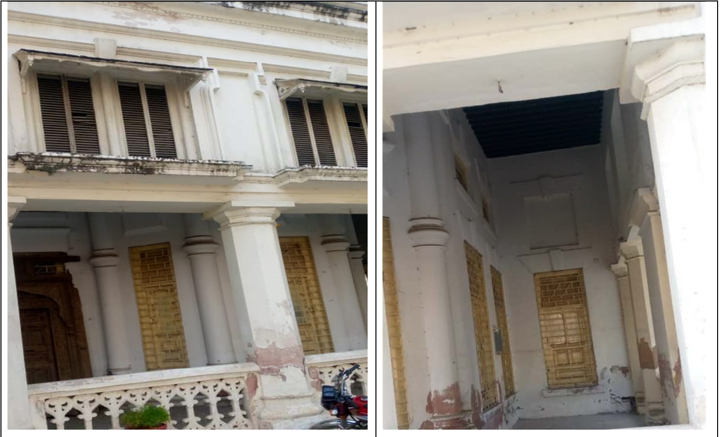
Figure 16. Construction Styles of the Building
