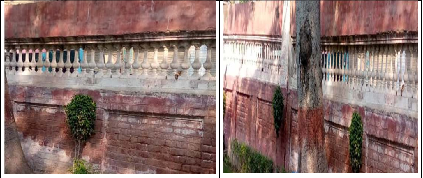
Figure 17. Construction Styles of the Building
