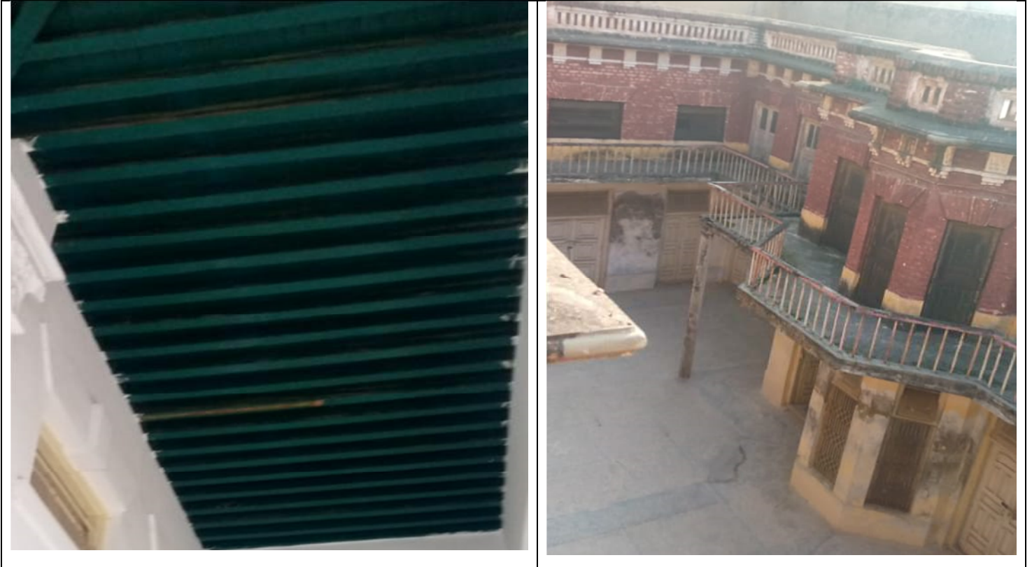
Figure 15. Construction Styles of the Building
